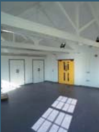
(Left) The refurbished Mercury Newspaper building for Cinderford Artspace. (See page 8).
